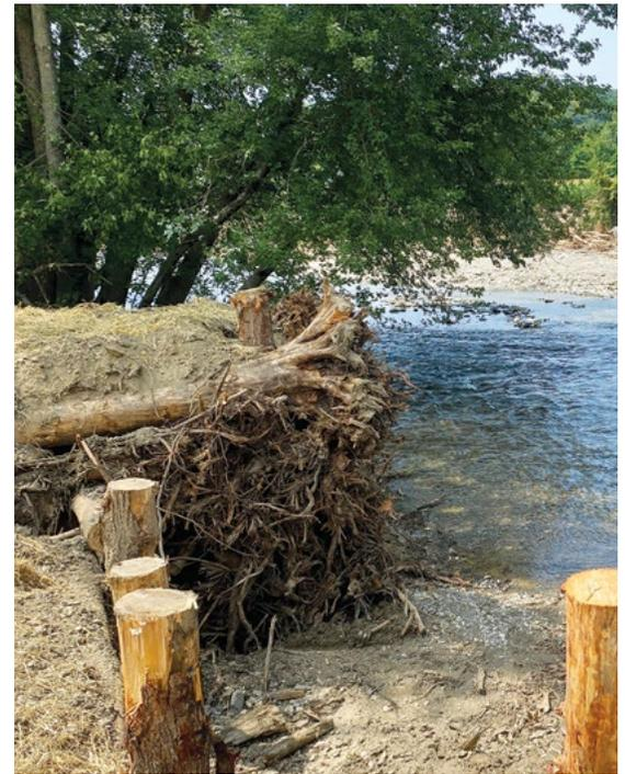
Rootwads are placed along the edges to direct the streamflow away, thus reducing erosion and naturally restoring the riverbanks.
