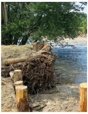
Rootwads are placed along the edges to direct the streamflow away, thus reducing erosion and naturally restoring the riverbanks.
